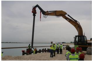
**Velana International Airport, Maldives 31st July 2017**— After the completion of all reclamation works today starts the official sheet piling works at Velana International Airport. Approximately 3,300 meters of sheet piling works at the north east lagoon area will be laid to protect the 650,000 square meters of land for the development of the new runway.
